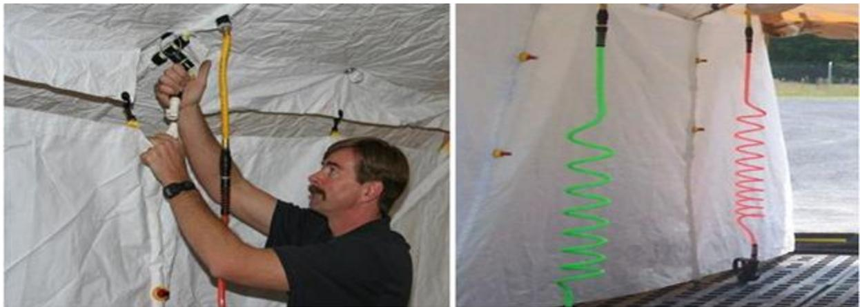
**Step 5.** Check with your Fire Department/CE Utilities if your installation requires a backflow device prior to connecting any fire hoses. Connect the water heater to a fire hydrant using a fire hose and a 2.5–1.5 inch adapter as shown in [Figure A3.22](#). Be sure to flush the hydrant before connecting it to the water heater. Normally, the water heater should be positioned on the clean side of the shelter for easier operation.
