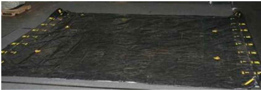
**Step 4.** Move the shelter bag to the corner of the berm where the inflator can be used. ([Figure A3.32](#)). It is best to have the corner downslope (if applicable) to ease the recovery process. This step requires four people.
