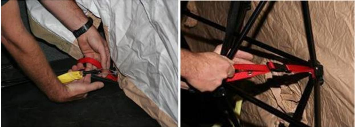
**Step 11.** When the red outer straps are secure, lower the lifting poles and secure to the sides of the shelter as handrails (**Figure A3.15**).
